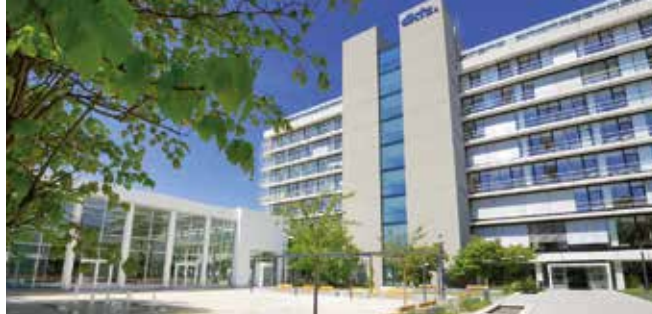
DKFZ main building (© Tobias Schwerdt / DKFZ)
